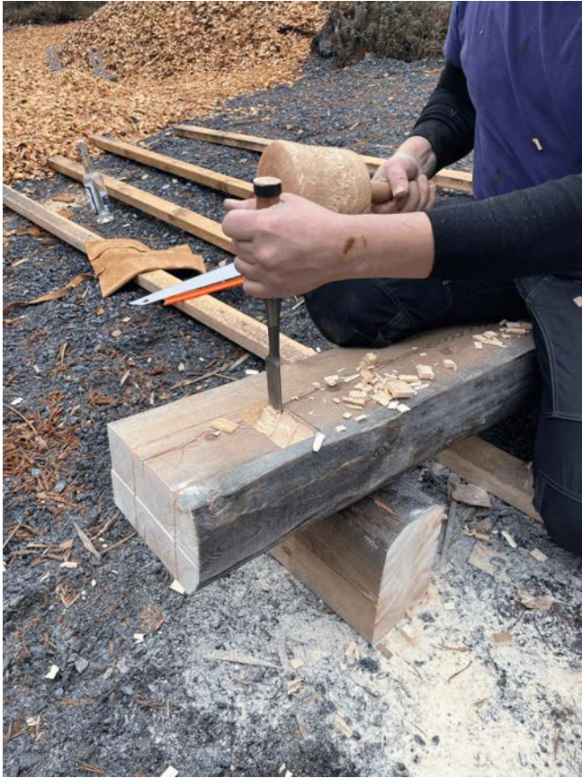
Making of a joinery. Most of the joints were tighten with a big pin.
