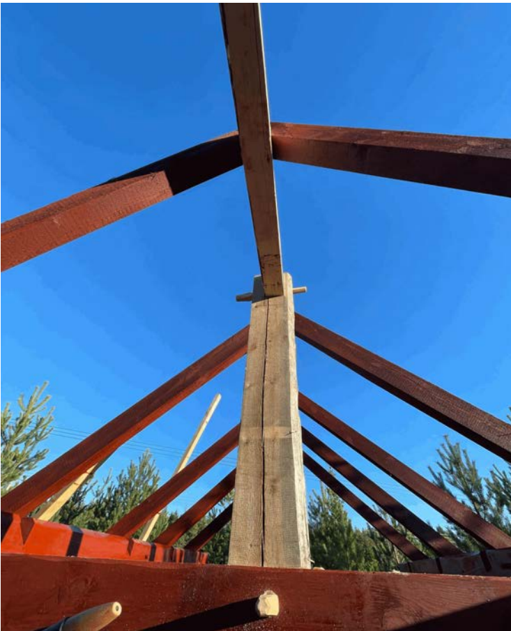
Making of a joinery. Most of the joints were tighten with a big pin.
